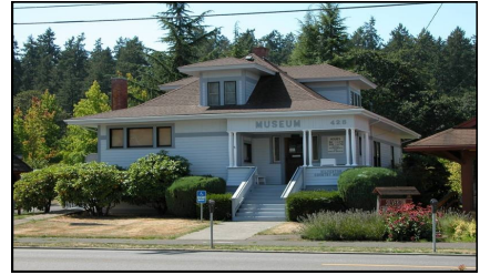
Museum and Office 428 South Water Street
