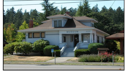
Museum and Office 428 South Water Street
