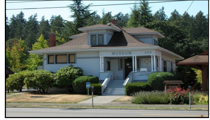
Museum and Office 428 South Water Street
