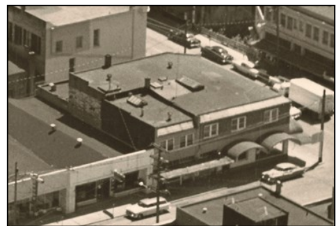
Worden building showing changed footprint
