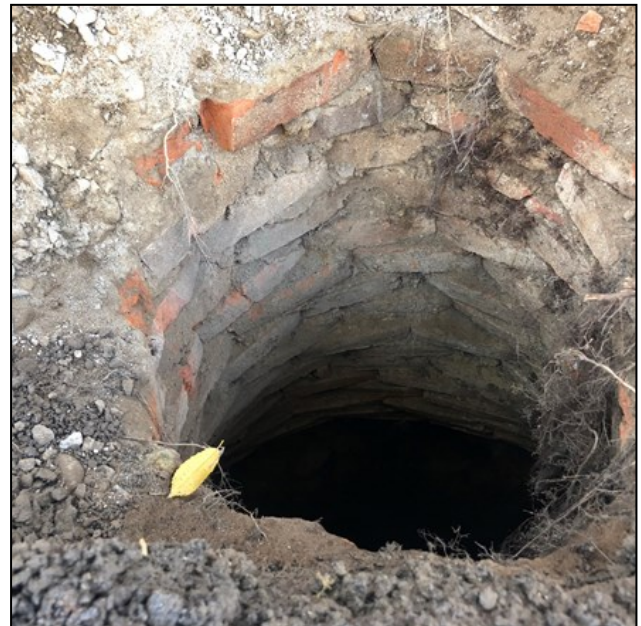
Early Silverton well on N. Water St. showing brick lining (Thanks to Ben Johnston for use of the photo)
