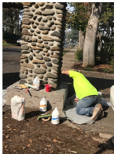
At long last the deteriorating condition of the arches is being addressed. After a thorough power washing to remove dirt and moss build up, new stones have been added and the mortar is being replaced and reinforced. They are looking amazing!
