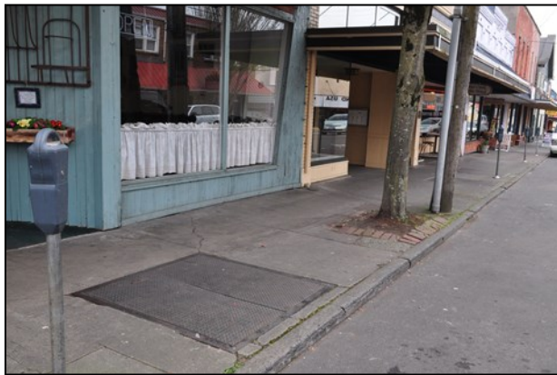
Doors at 105 N. Water before removal
