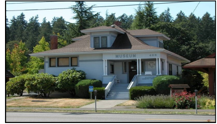
Museum and Office 428 South Water Street
